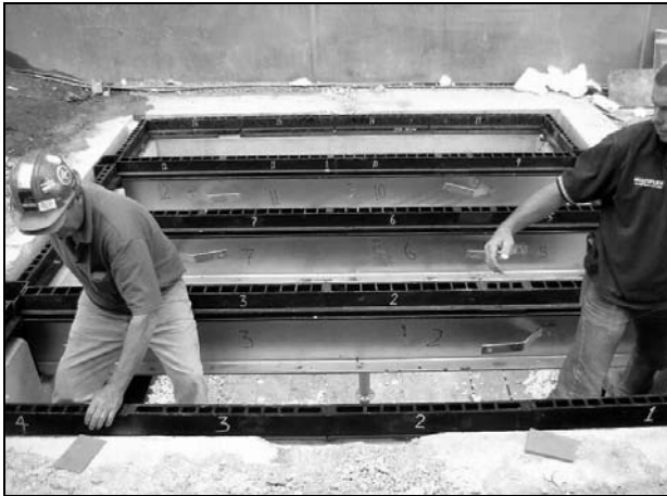
Figure 2 – Frame Sections & Beams are Numbered
